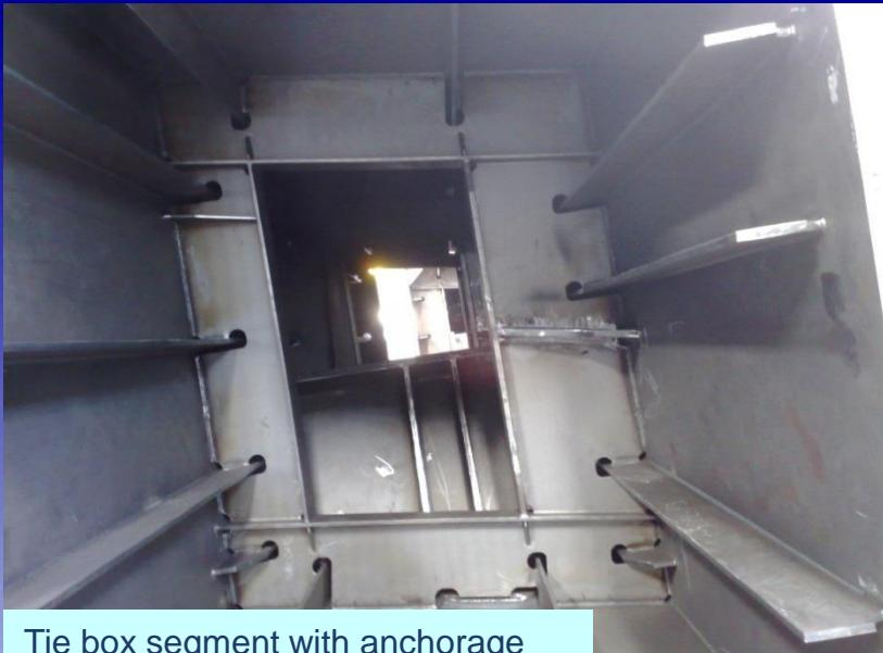
Tie box segment with anchorage structure
